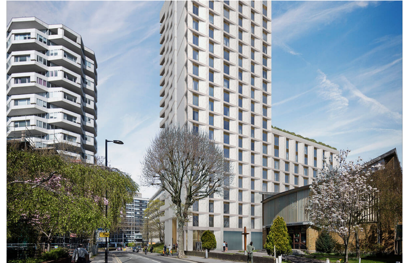
Addiscombe Grove, Croydon – Optivo's joint project with Pocket Living
